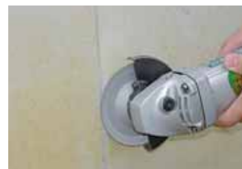
▲ For eliminating difference in level on concrete walls
