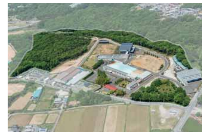
Overview of head office
